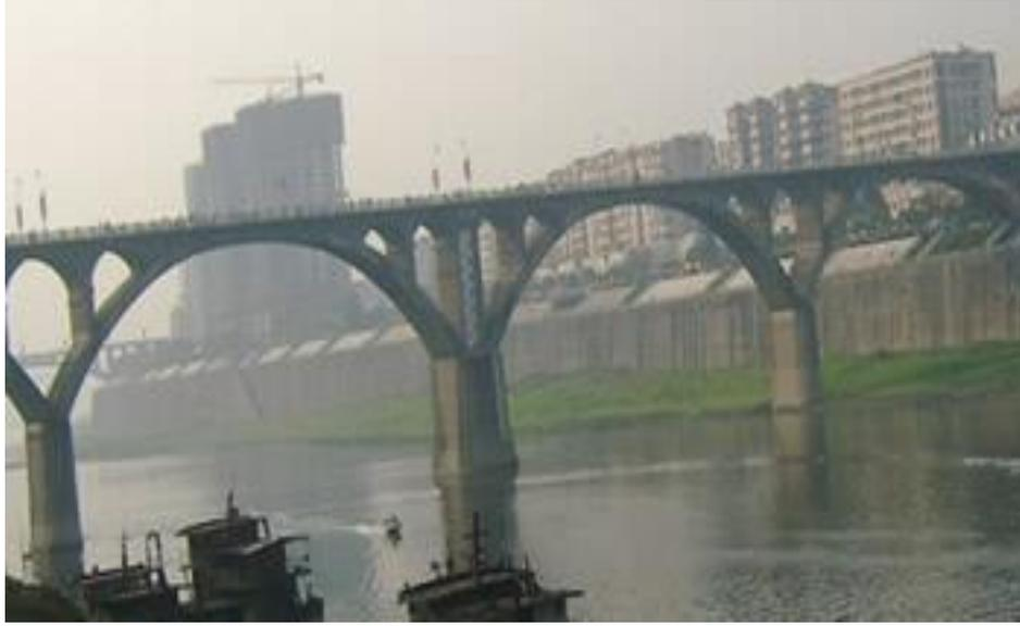
An arch bridge: a parabola represents the profile of the supporting structure of an arch bridge. This concrete bridge transfers its weight horizontally into abutments
