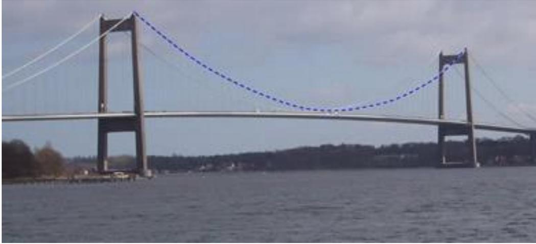
**A suspension bridge: a parabola represents the profile of the cable of a suspended-deck suspension bridge. The curve of the cable created by the chains follows the curve of a parabola.**
