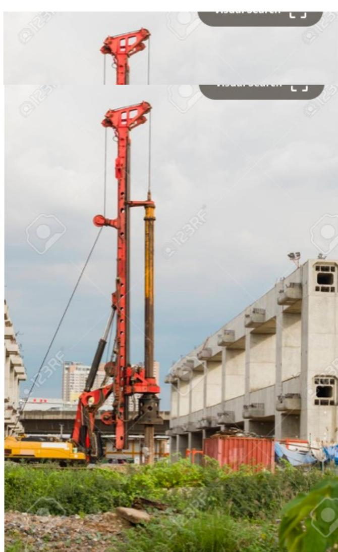
bored pile machine, dry process
