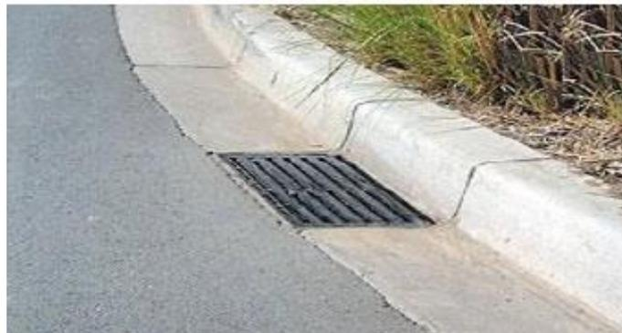
**Figure 2.6: Cutter drainage system**
