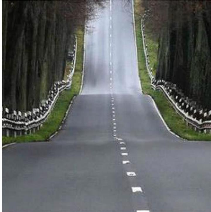
Two basic types of vertical curves exist, crest and sag. Crest type undergoes a negative change in grade; that is, the curve turns downward. Sag type undergoes a positive change in grade; that is, the curve turns upward. There are several factors that must be taken into account when designing a grade line of tangents and curves on any highway or railroad project. They include:
