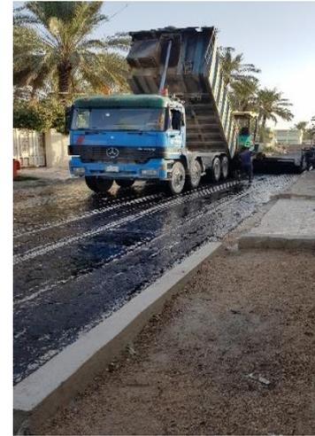
c. **Rapid-Curing asphalt (RC)**: RC asphalts are produced by blending asphalt cement with a petroleum distillate that will easily evaporate, such as **Gasoline or naphtha**. RCs are used as a tack coat between the binder and wearing course.
