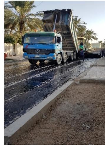
c. **Rapid-Curing asphalt (RC)**: RC asphalts are produced by blending asphalt cement with a petroleum distillate that will easily evaporate, such as **Gasoline or naphtha**. RCs are used as a tack coat between the binder and wearing course.
