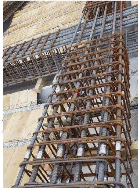
Figure 5: Details of shear reinforcement
