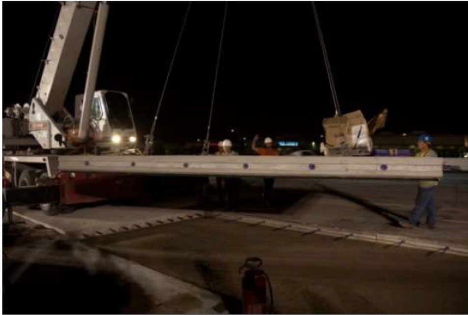
Figure 1. Full depth pavement replaced with PPCS.
