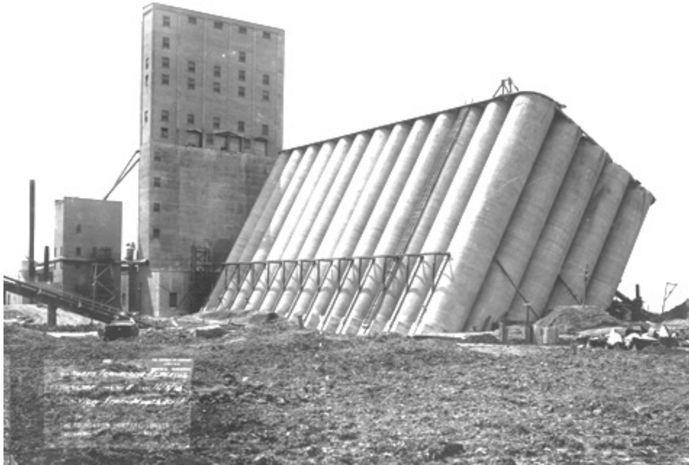
The tilted Transcona grain elevator (Courtesy: UMA Engineering Ltd., Manitoba, Canada)
