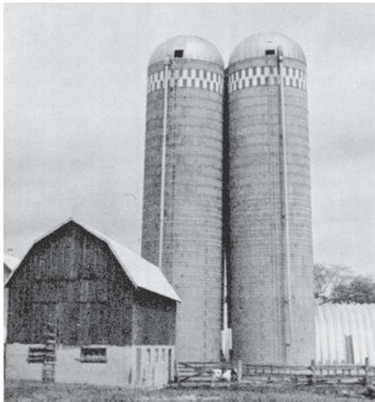
FIGURE 7.1 The “kissing” silos. (Bozozuk, 1976, permission from National Research Council of Canada.) These silos tilt toward each other at the top because stresses in the soil overlap at and near the internal edges of their foundations. The foundations are too close to each other.
