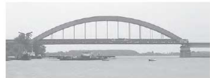
Arches support their loads in compression.
