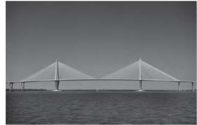
Cables support their loads in tension.
