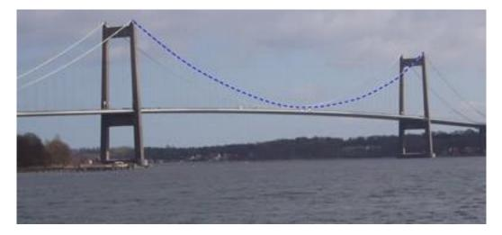
A suspension bridge: a parabola represents the profile of the cable of a suspended-deck suspension bridge. The curve of the cable created by the chains follows the curve of a parabola.
