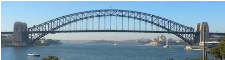
Long Span Steel Bridge
