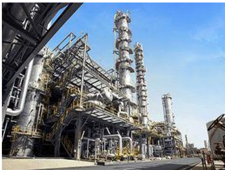
Petrochemical plant in the Kingdom of Saudi Arabia
