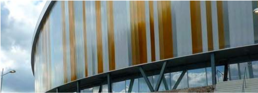
Rodeca Round Facade at Omnisport Arena Apeldoorn
