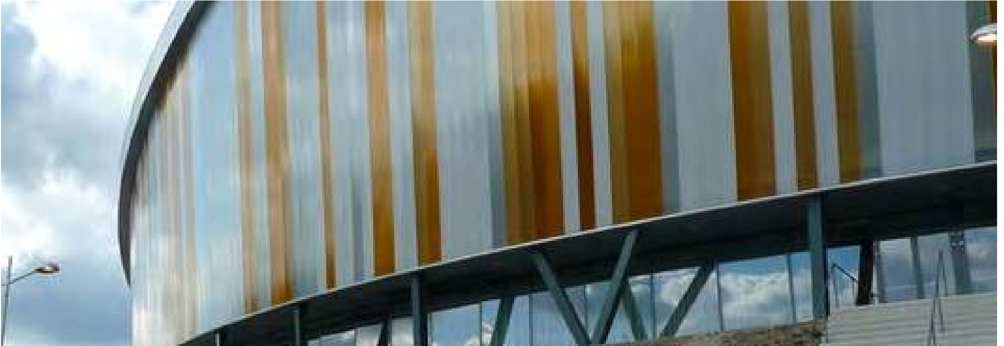
Rodeca Round Facade at Omnisport Arena Apeldoorn
