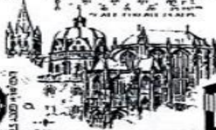
(F) EXTERIOR FROM SW.
