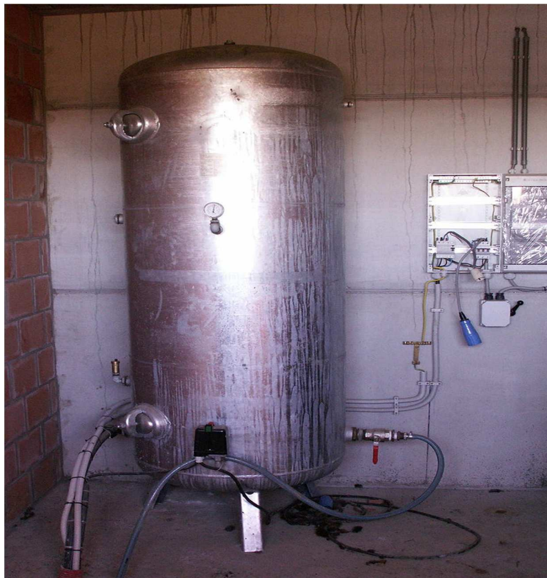
Fig.2 Pressurizing the water is required between the small water reserve and the end-user
