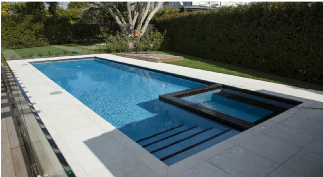
Fig.1 Concrete swimming pool
